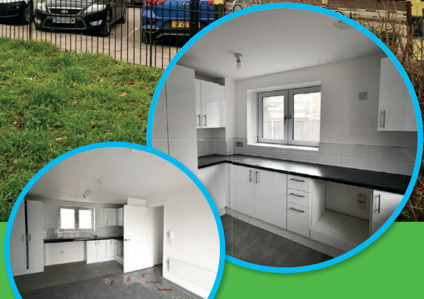
Building works in progress
